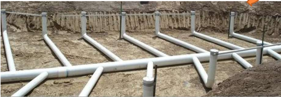
Sewell Reserve - Bioretention system © Clearwater, 2012
