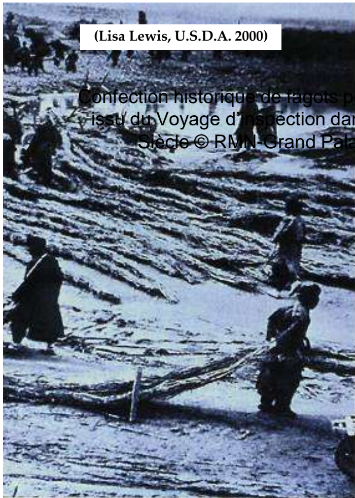
China Early 1900's. Bundling live stems for use in riverbank and dike repair. Kevin Finney
