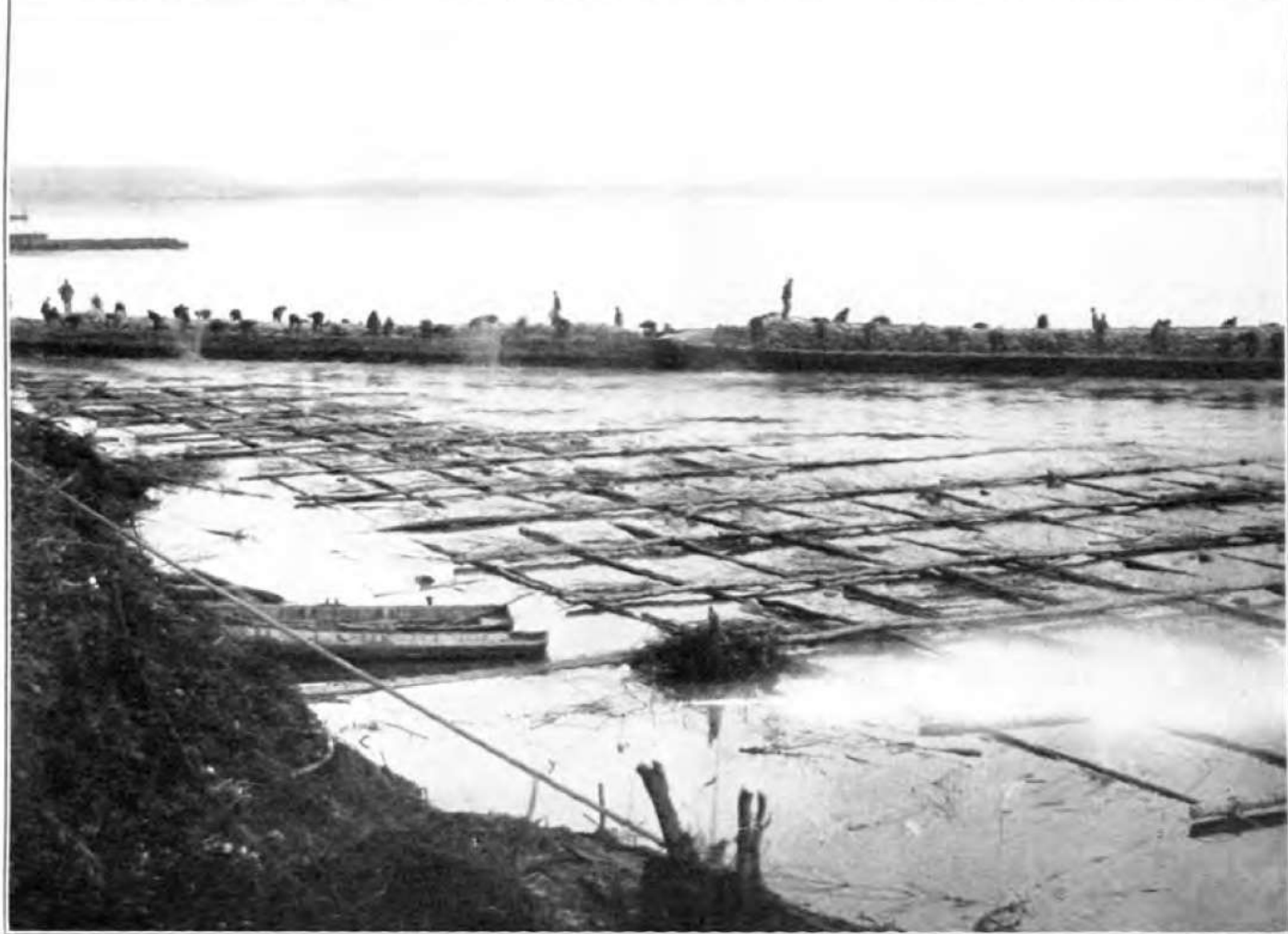
NO. 7.—SINKING SUBAQUEOUS MAT—CLOSE OF THE OPERATION.
