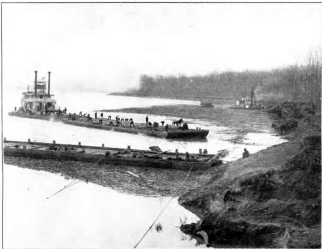
NO. 6.—SINKING SUBAQUEOUS MAT—SECOND STAGE.
